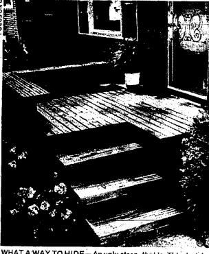
WHAT A WAY TO HIDE—An ugly stoop, that is. This deck is an example of a project you can build to cover a concrete stoop. It's entirely supported by a ledger anchored to the house and by three 4 x 4 posts. The understructure and skirt are made of 2 x 8s; the decking is 2 x 4s. For information on deck projects, send \$2 to Georgia Parific Corporation. The deck projects, send \$2 to Georgia Pacific Corporation, The Deck Book, Dept. M, P.O. Box 48408, Atlanta, Ga., 30362.
