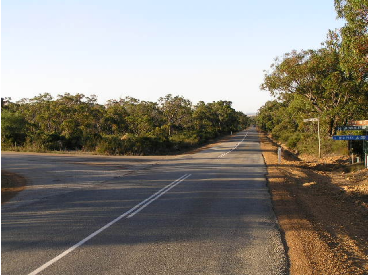
PLATE 9 – View showing vegetation on northern side of Formby South Road (facing north) from Albany – Lake Grace Road. It appears that that there is partial revegetation of an old stockpile site on this northwest corner of the intersection with the heritage plaque (Refer Plate 10) also located on this site. Fishtail widening is required on this corner.
