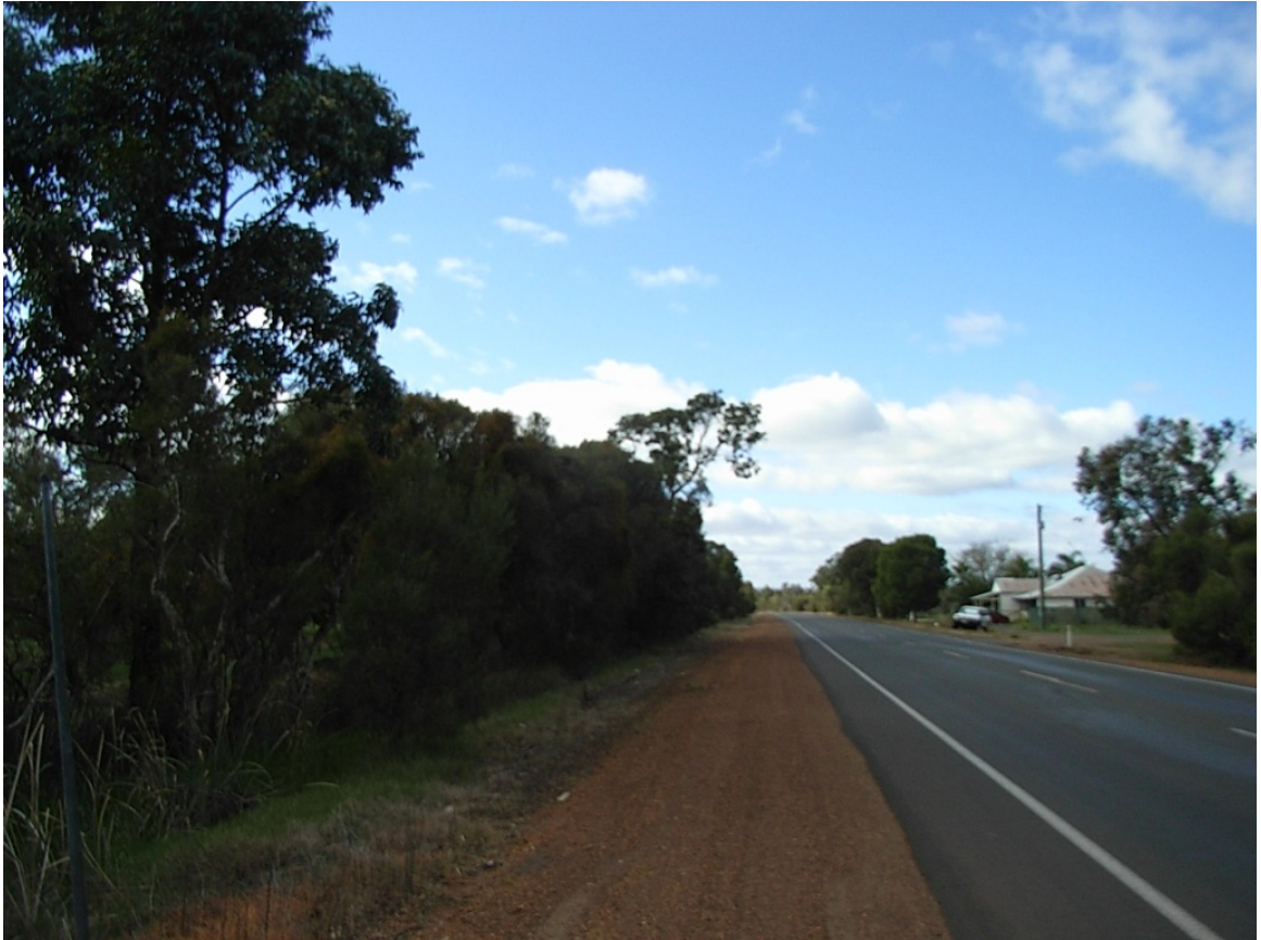
Photo 6: View north east showing proximity of the closet residence at 144.10 SLK – clearing on left side
