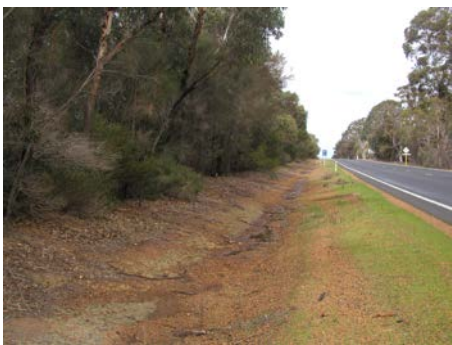
H1 Oconnor Rd area "Soft Verge"
