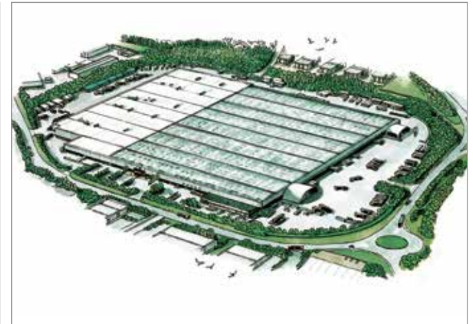
National Distribution Centre - Northampton
