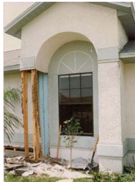
Fig 14-15 – A tunnel in the wood (left) and a great building damage of Subterranean termites (right).
