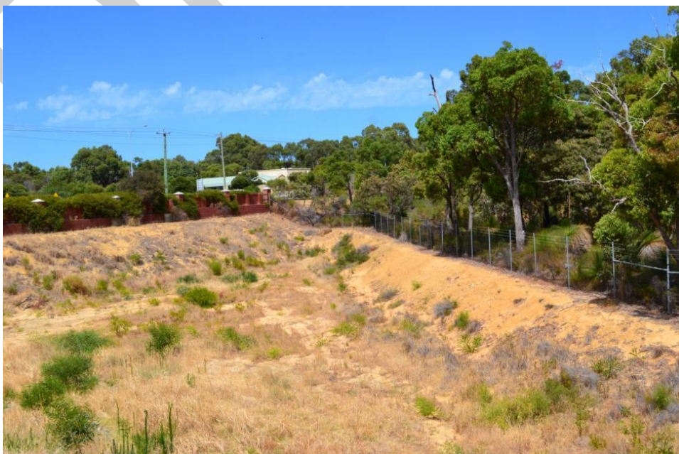
Figure 27: Fenced off Sump at Hepburn Heights
