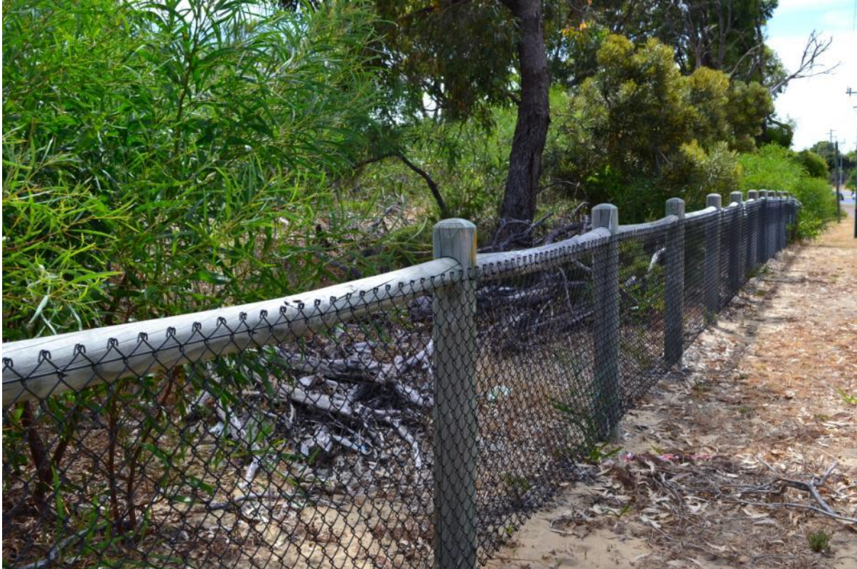
Figure 24: Conservation Fencing on the Perimeter of Hepburn Heights
