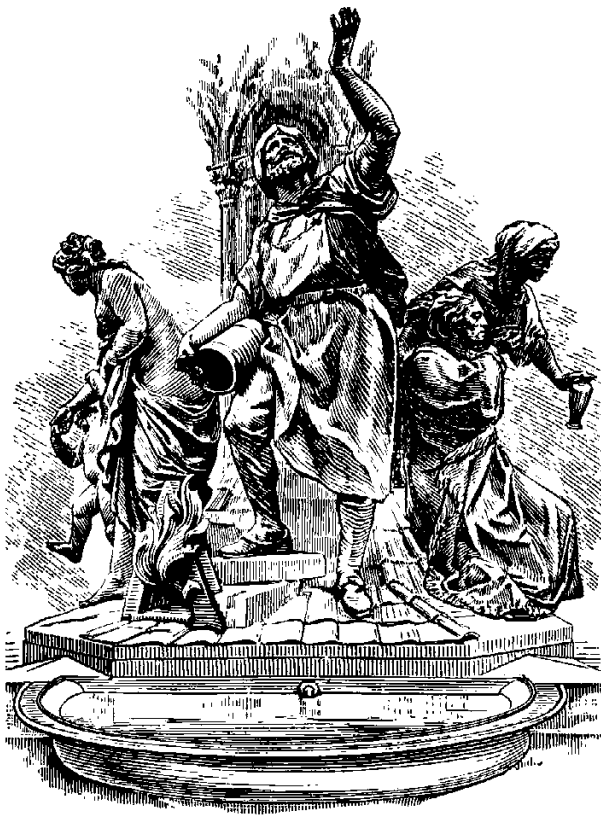
GROUP ON FOUNTAIN—NORTH.
