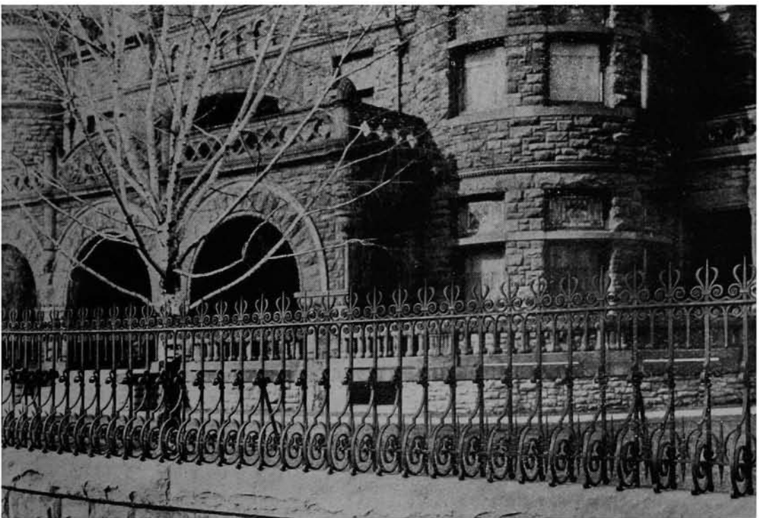
Hand Forged Wrought Iron Railing.
