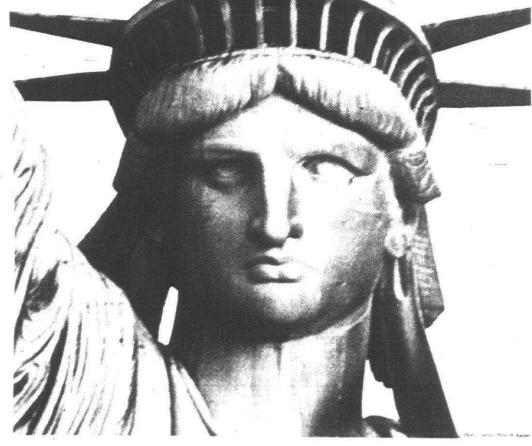
For nearly a hundred years, the Statue of Liberty has been America's most powerful symbol of freedom and hope. Today the corrosive action of almost a century of weather and sollution has eaten away at the iron framework. etched holes in the copper exterior.
