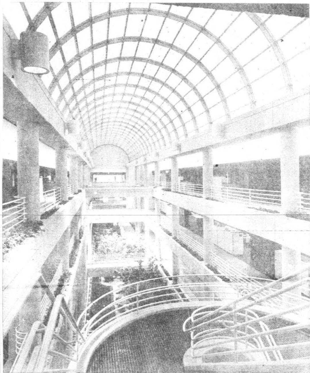
The office block of the Comerica Operations Center is bisected by a 30-foot-wide, four-story skylit atrium, which allows daylight to penetrate deep into the building.
