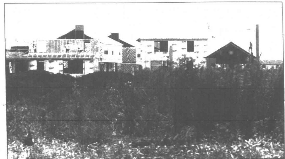
Homes are in the construction phase on Beck Road between Warren and Ford roads.
