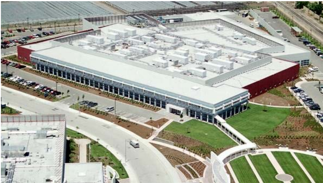
Bldg. 10 R&D facility on 1710 Automation Parkway, Milpitas, CA built in 1997.
