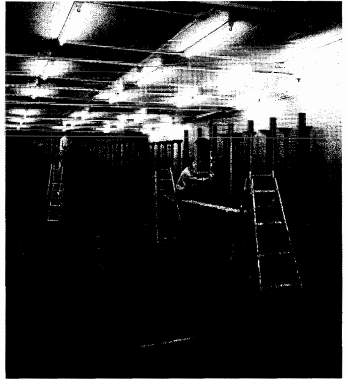
Computer room construction
