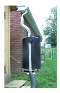
Please read the Disclaimer on the inside cover, if you are interested in installing this project. rain barrel collects and stores stormwater runoff from rooftops. By detaining (temporarily holding) the stormwater runoff during a rain event, you can help add capacity to the city's sewer system and reduce sewer overflows to our creeks and rivers, our drinking water source. Also, the collected rain water can be reused for irrigation to water lawns, gardens, window boxes or street trees.
