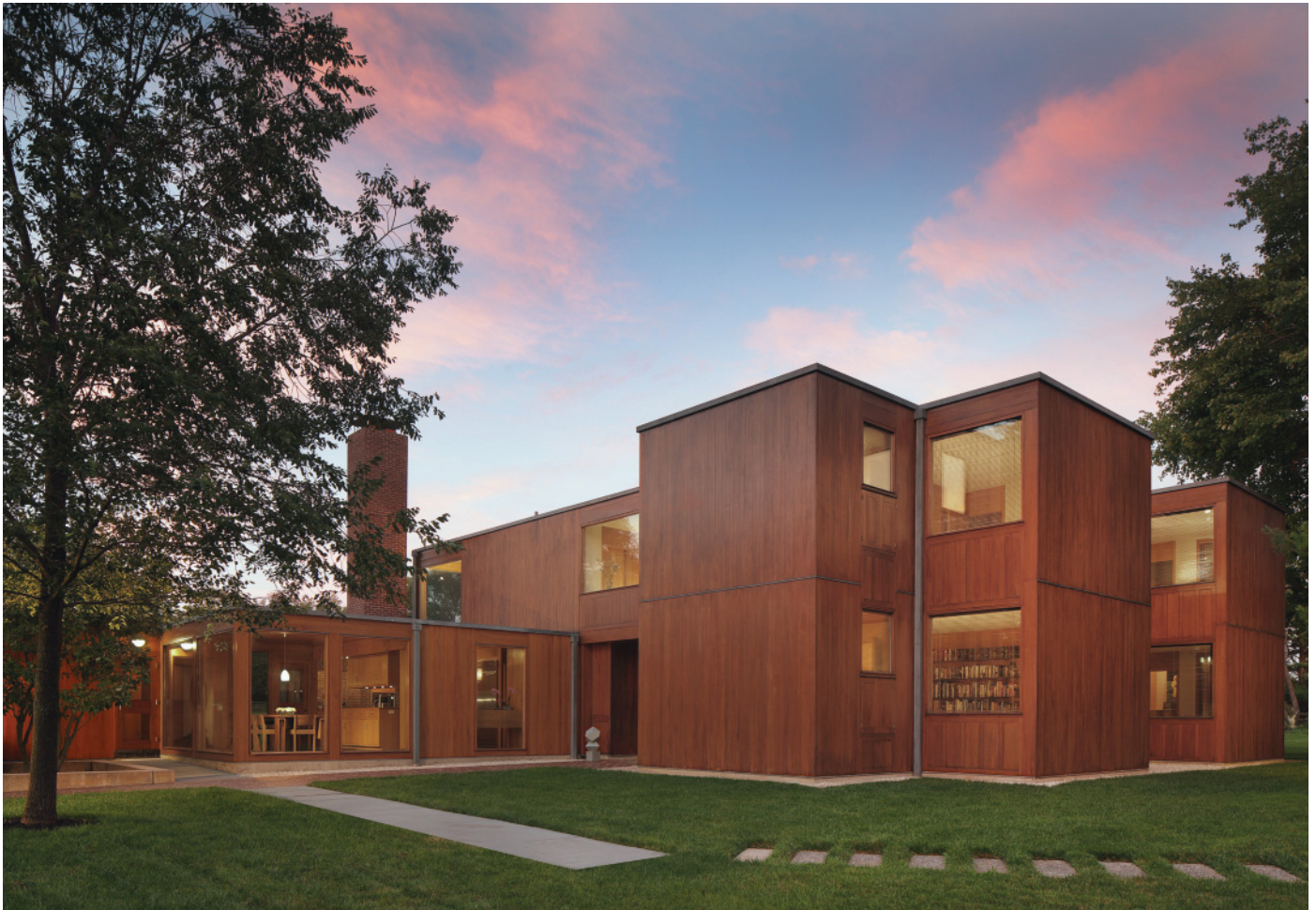
Fig. 5. Korman House, before treatment, 2014
