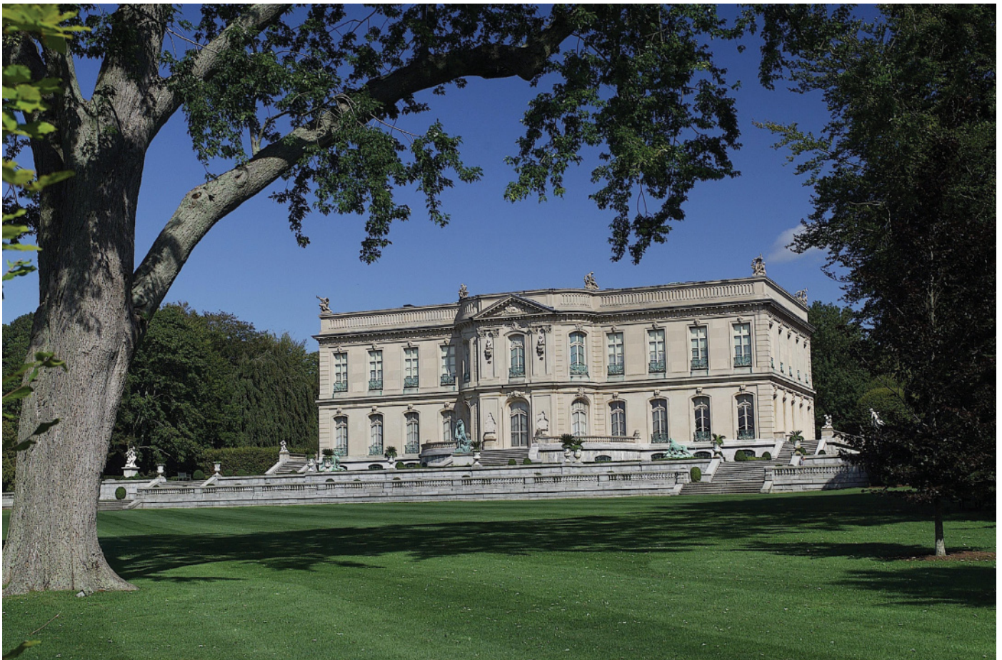
Fig. 1. The Elms (1901), West façade
