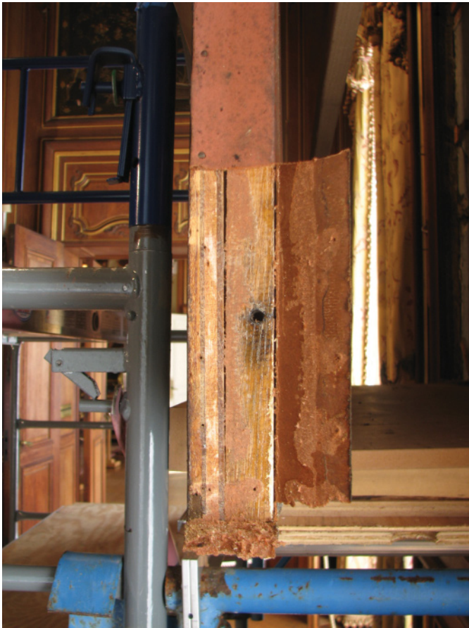
Fig. 8. Wood laminations are visible on the edge of the West panel.
