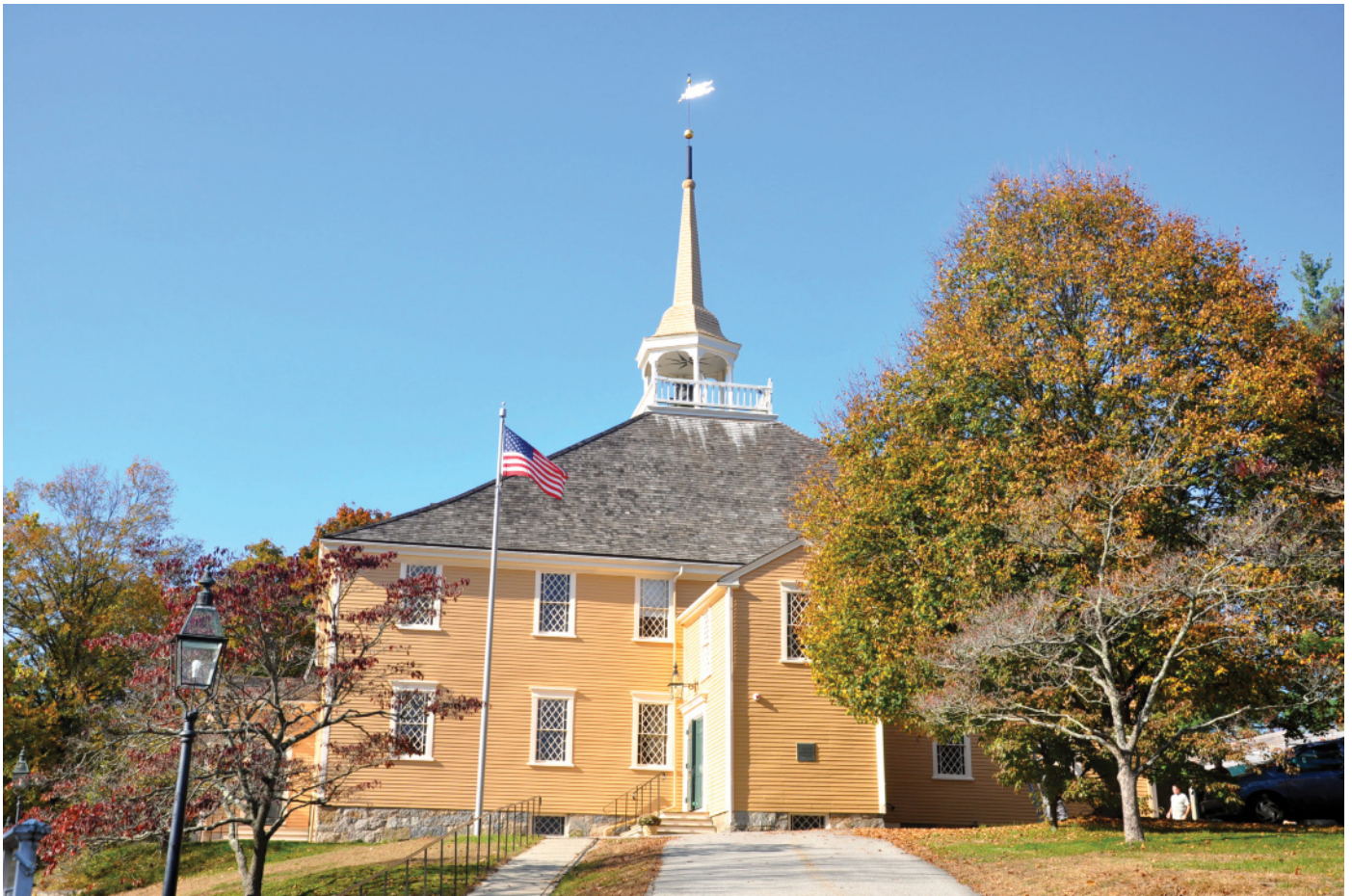
Fig. 1. Exterior view of Old Ship Church, south façade, 2014 (Courtesy of Building Conservation Associates Incorporated)
