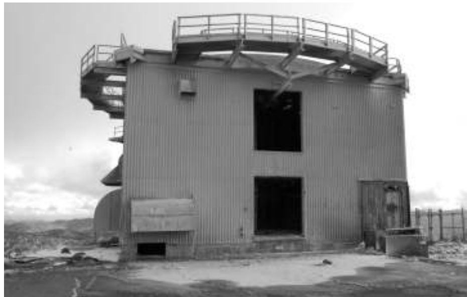
Structure at abandoned Air Force base, Mount Laguna
