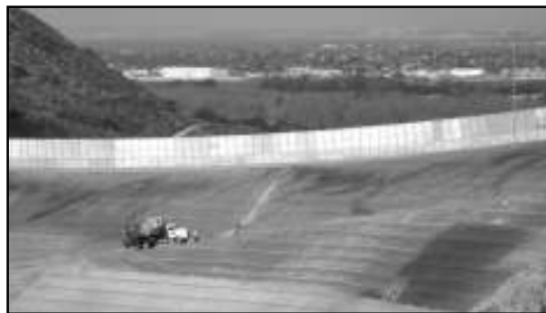
Secondary fence crossing Smuggler's Gulch; San Diego in background
