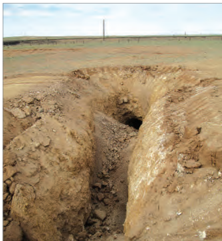
Technical infilling underway
