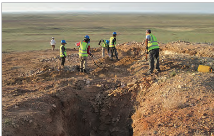
Manual approaches also necessary to distribute topsoils
