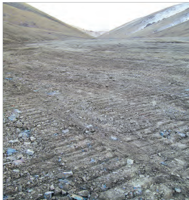
2. Compaction at non-FRD rehabilitation area, Jargalant October 2014
