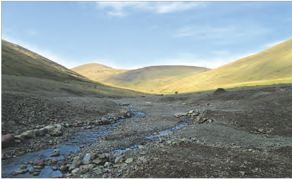
Technical rehabilitation almost complete
