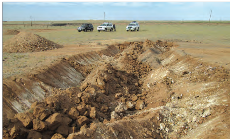
Mechanized infill almost complete
