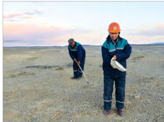
Sowing and raking selected seeds into topsoils
