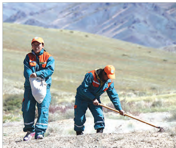
Sowing and raking seeds into topsoils
