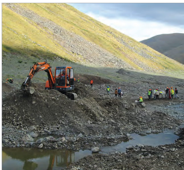
A light excavator was used for technical rehabilitation
