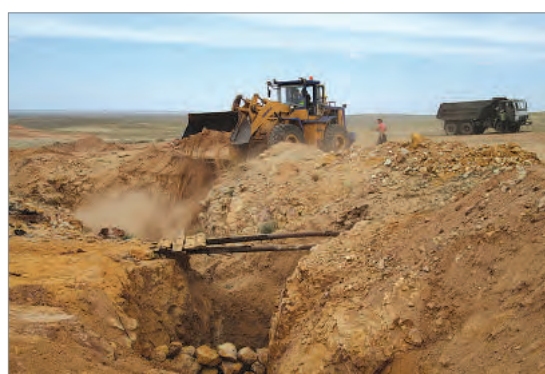
Mechanized infill was necessary
