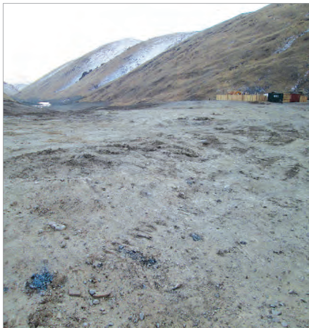
1. Mechanized compaction at non-FRD rehabilitation area, Jargalant October 2014
