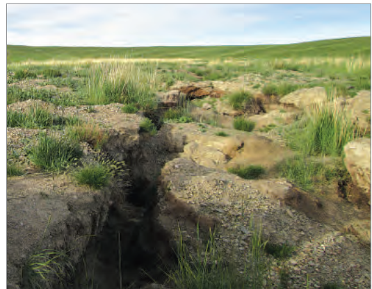
Conditions before rehabilitation
