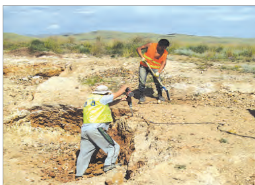
Reprofiling required hand drills
