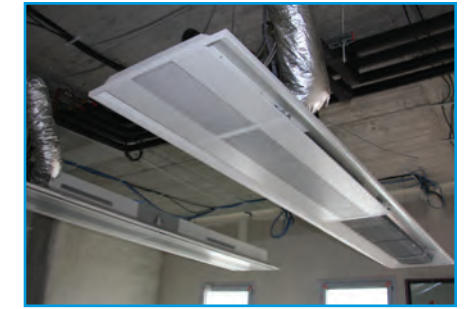
Chilled beams
