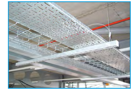
Multiple cable trays on single channel
