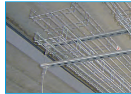
Multi-tiered cable basket on Trapeze
