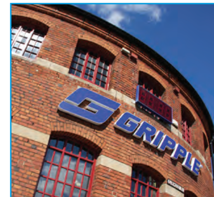
The Old West Gun Works, Sheffield, UK
