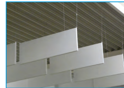
Acoustic baffles
