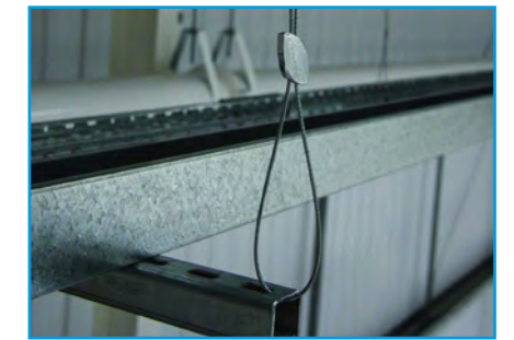
Perforated cable tray on channel
