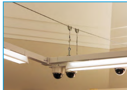
Lighting and Camera on Catenary
