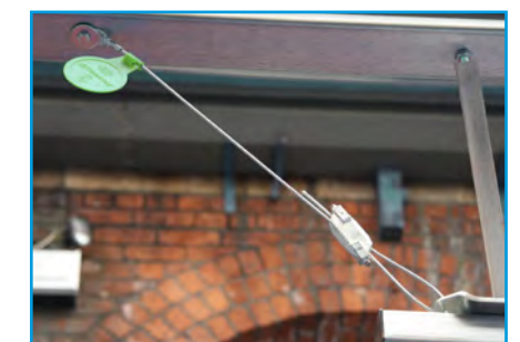
Transverse Bracing
