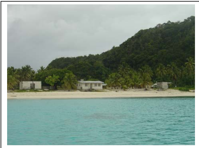
Coastal erosion is a major problem for the Naikaleyaga villagers as it threatens infrastructure such as the school and medical center
