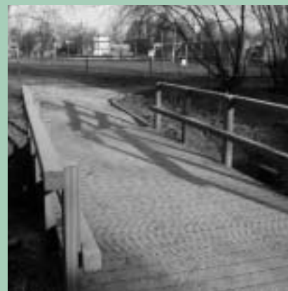
A bridge made of FSC labelled wood in the municipality of Edegem
