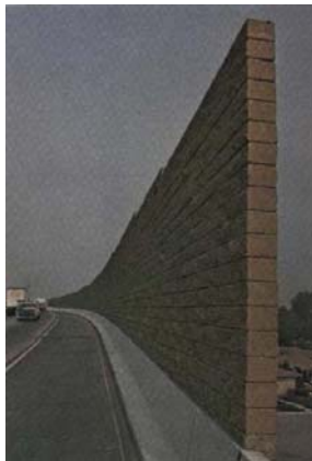
Fig. 12. Abrupt endings on wall
