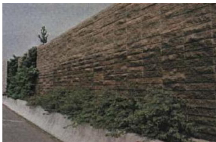
Photo 75. A wall which varies in plan view, to reduce the straight line effect, and provide visual interest
