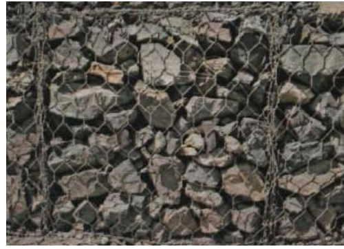
Photo 77. Gabions are essentially wire baskets filled with stone
