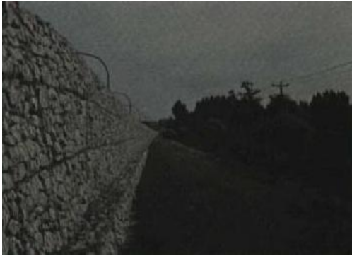
Photo 76. A gabion noise wall
