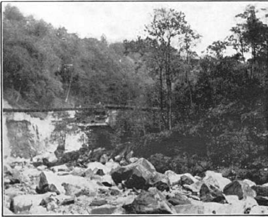
RAILWAY BRIDGE IN ARNCLIFFE WOODS AFTER FLOOD IN JULY, 1930.
