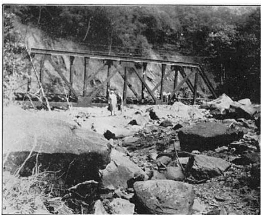
NEW RAILWAY BRIDGE IN ARNCLIFFE WOODS, AS DESTROYED BY THE FLOODS IN SEPT., 1931.
