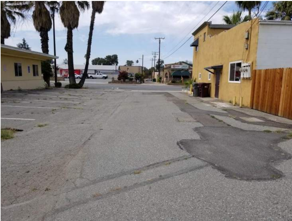
Photo 2: Egan Alley Project Site (S)
