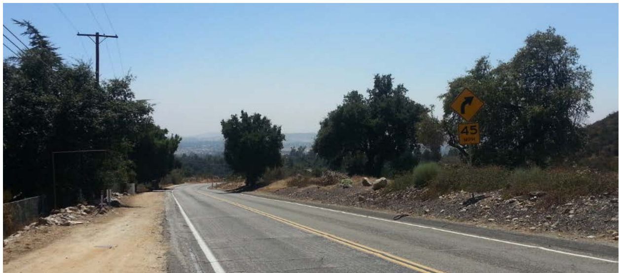
Photograph No. 2: Present alignment condition along Oak Glen Road (Pipeline 2)
