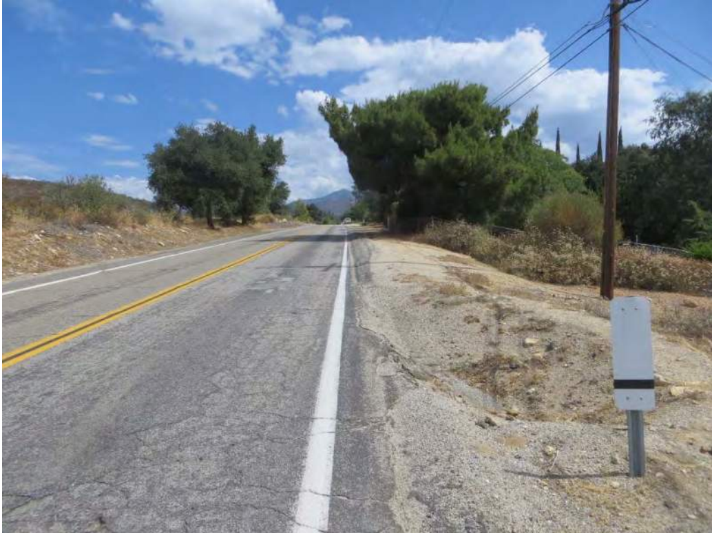
Photograph 8: View of the proposed pipeline location along Oak Glen Road within the southern portion of the Apple Tree Lane Survey Area, facing north.
