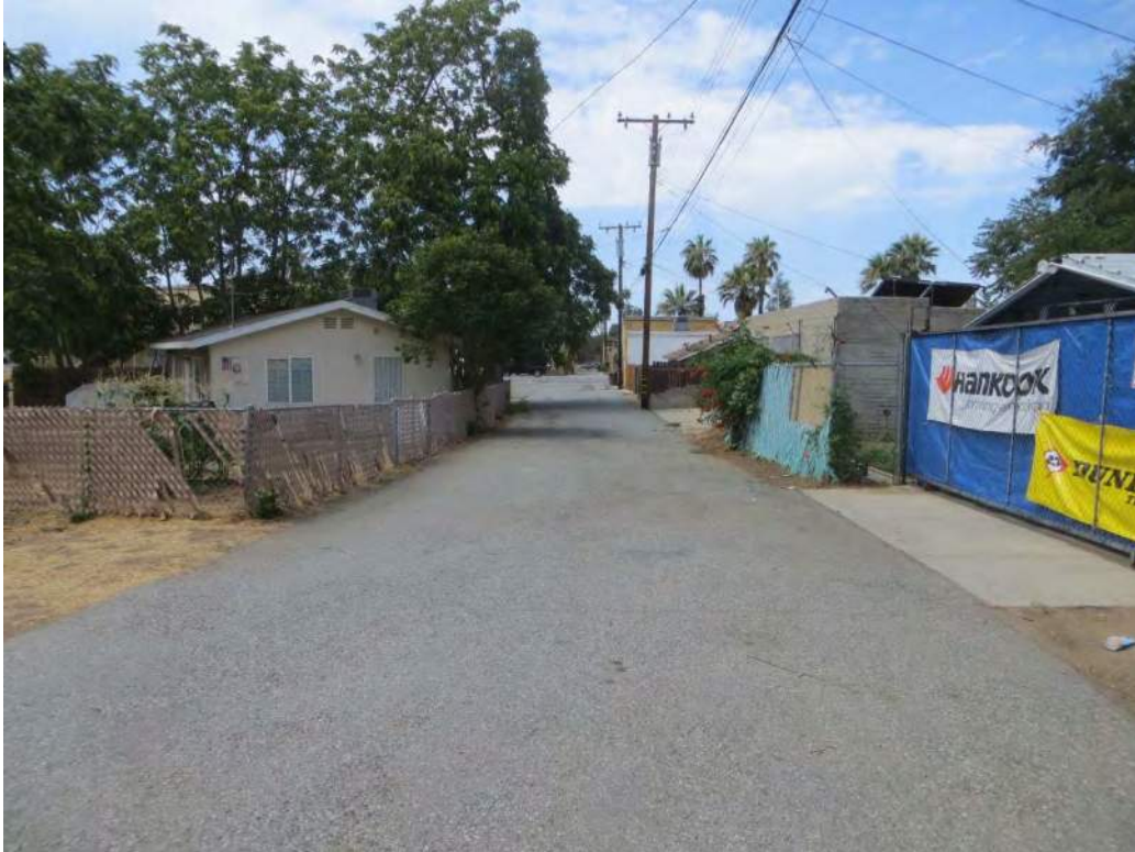
Photograph 10: View of the proposed pipeline location within the northern portion of the Egan Alley Survey Area, facing southwest.
