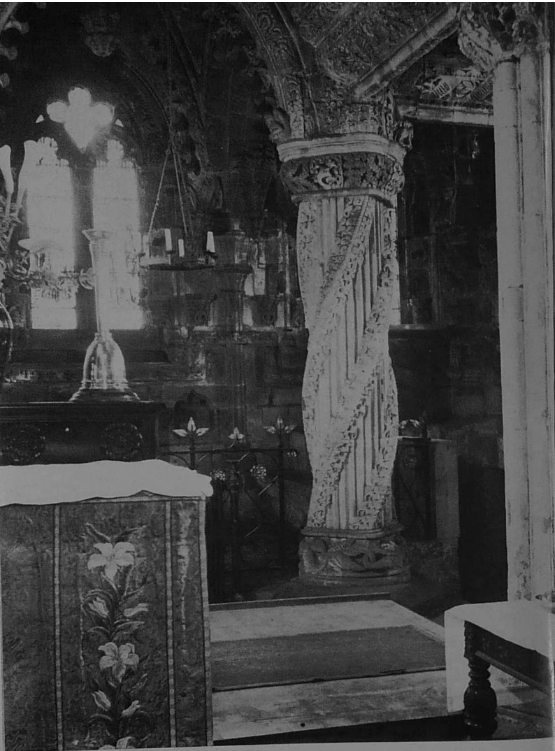
Plate 10 The Prentice Pillar (Roslin Chapel, Midlothian). Fifteenth century
