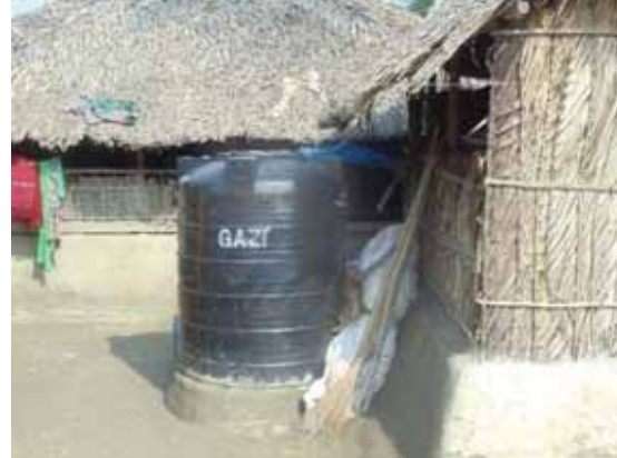
Photo 6.10: Domestic Level Rain Water Harvesting
