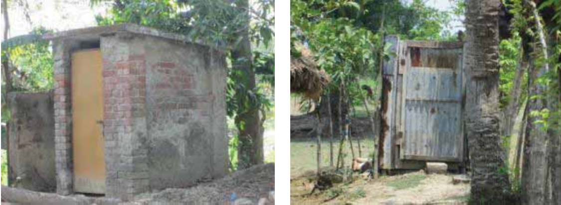
Photo 6.7: Sanitation Facility in the Polder Area
