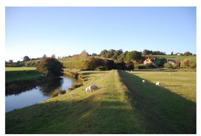
**Typical example of a flood** embankment
