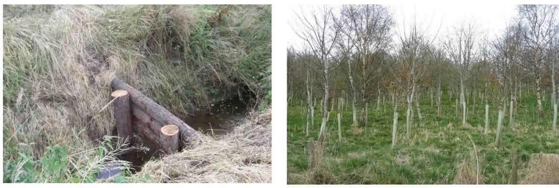
**Typical example of in**channel debris barrier
