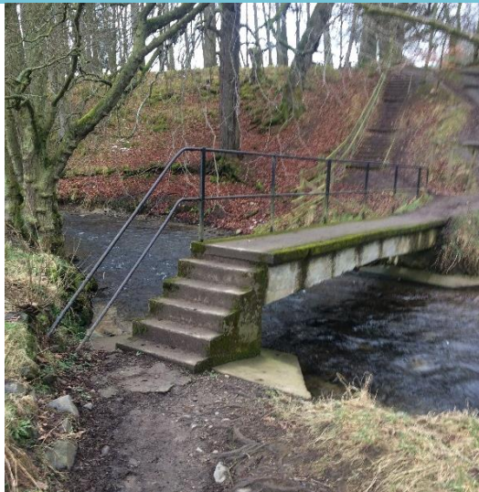
Concrete bridge spanning Haystoun Burn
