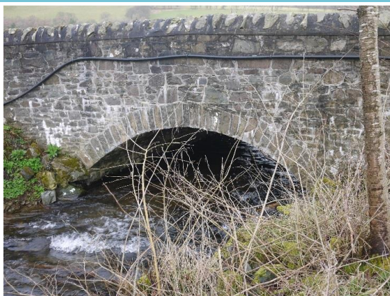
Upstream face of bridge
