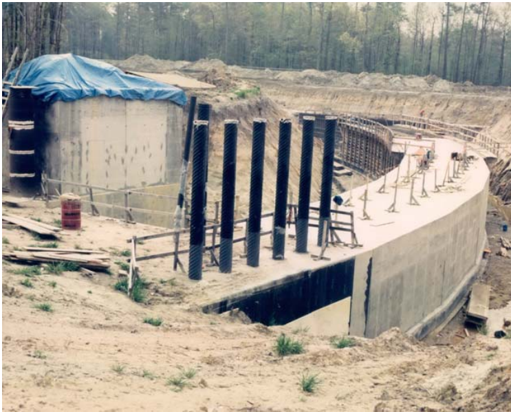
East Arc Tunnel
