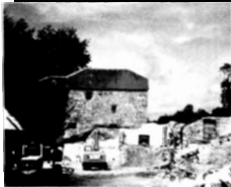
Work in progress at the Clashganny Mills project.
