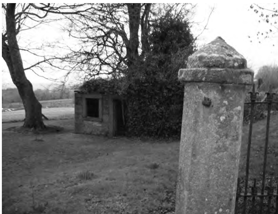
Gate Lodge at Woodside House, Hacketstown, formerly owned by the Jones family
