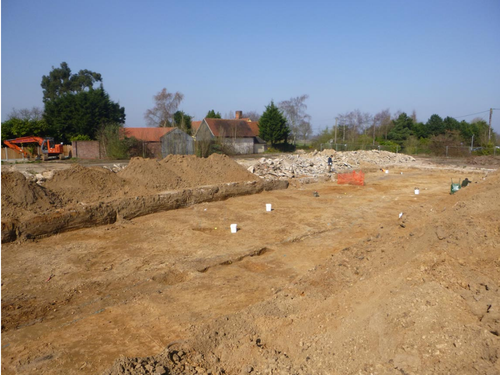
Photograph 1 Excavation area 1, looking N
