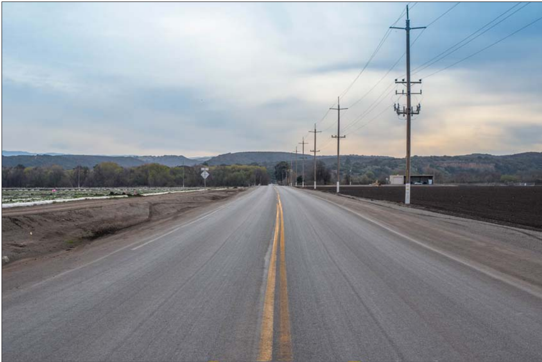
Figure 2.7-3a: Viewpoint 2, Near Proposed Bridge Site Looking Southwest, Existing View
