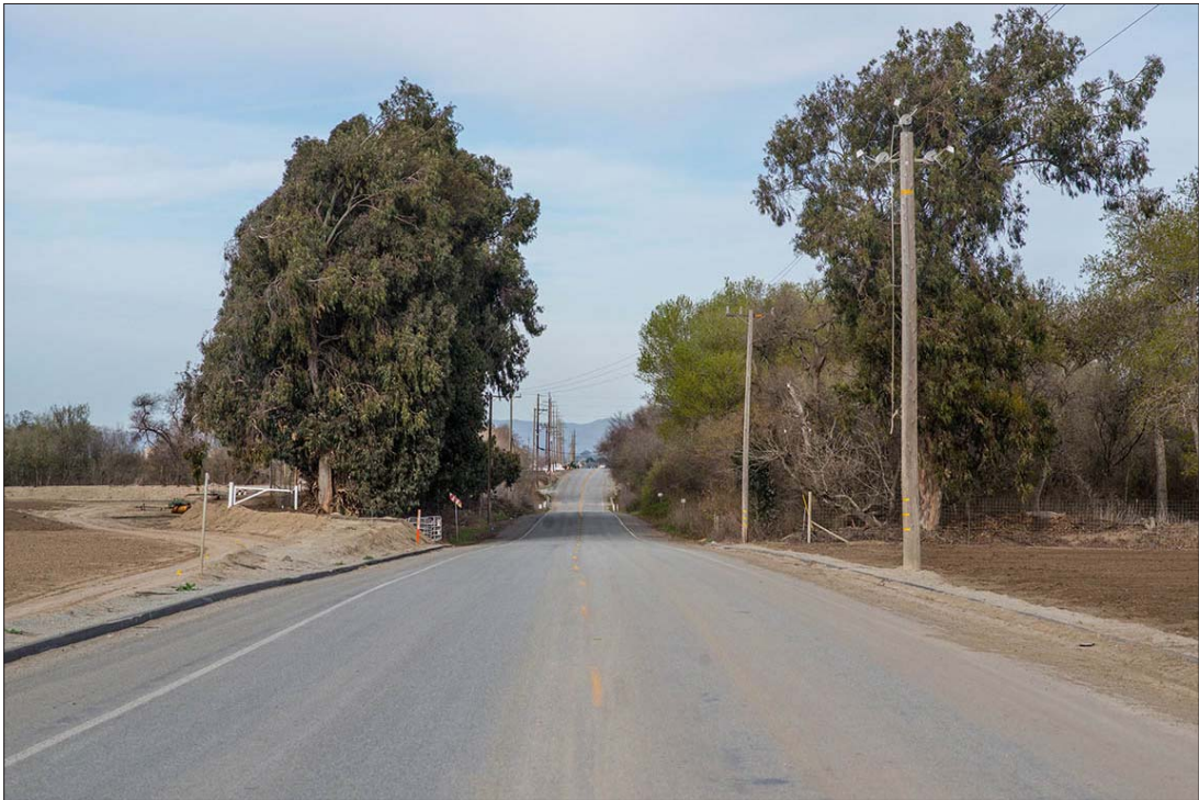
Figure 2.7-4a: Viewpoint 3, Near Proposed Bridge Site Looking Northeast, Existing View
