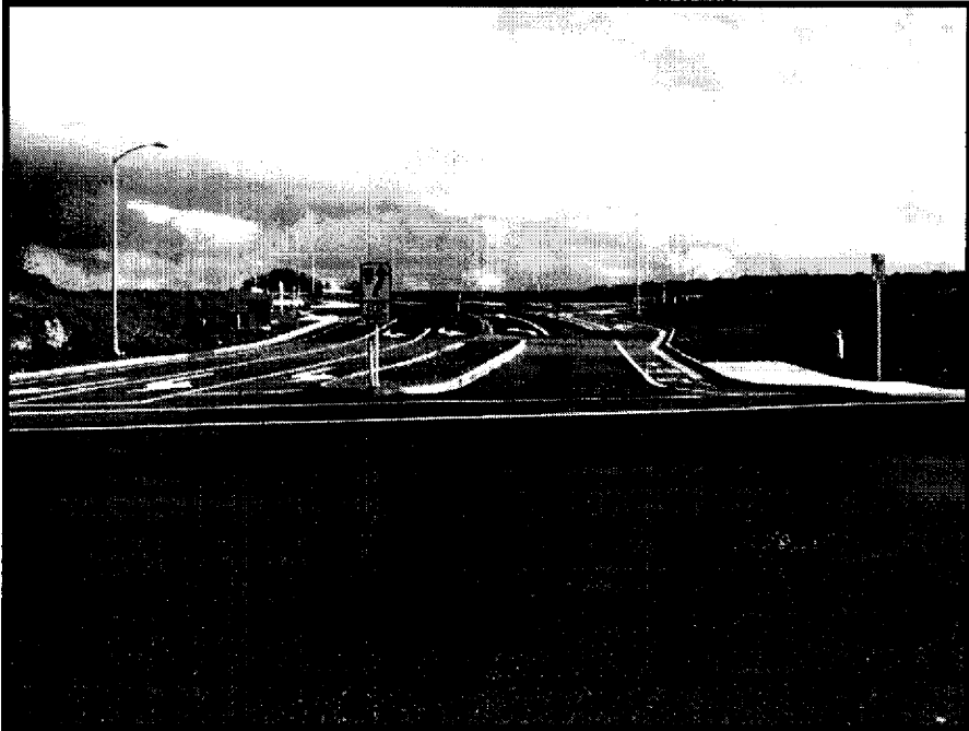
Stone Point Drive facing east from North Sunrise Avenue
