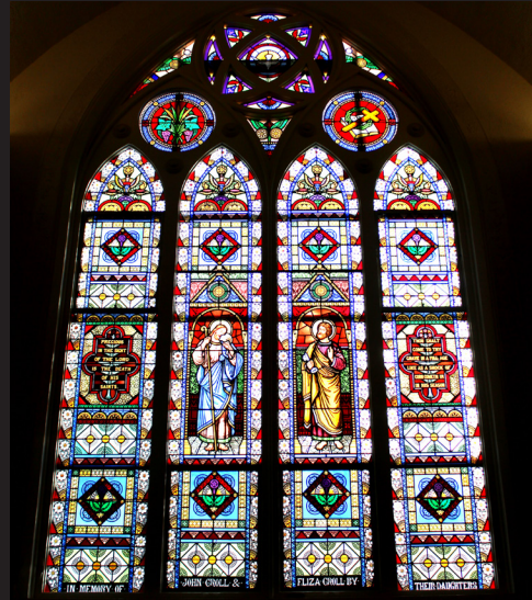
New lighting makes the front stained glass window at the church glow at night.
