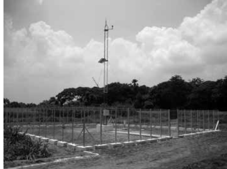
AWS installed by IMD at Madhavaram, Chennai
