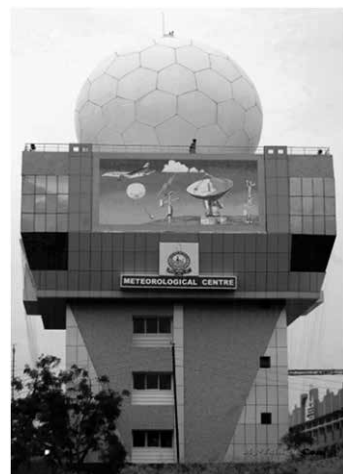
The S-Band Doppler Weather Radar installed at Hyderabad in 2010
