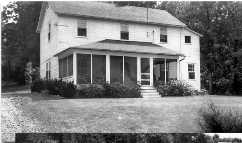
(Left) A photograph of the former WB&HIC “bunkhouse” (and formerly occupied by foreman Harry Lawson and family) taken in August 1959 records the addition of a screened-in porch by Wilkes-Barre attorney George Fenner Jr. and his wife Hilda, for whom the converted lakeside dwelling was serving as a summer cottage. An arsonist would reduce this building to ashes on the morning of February 15, 1989.
