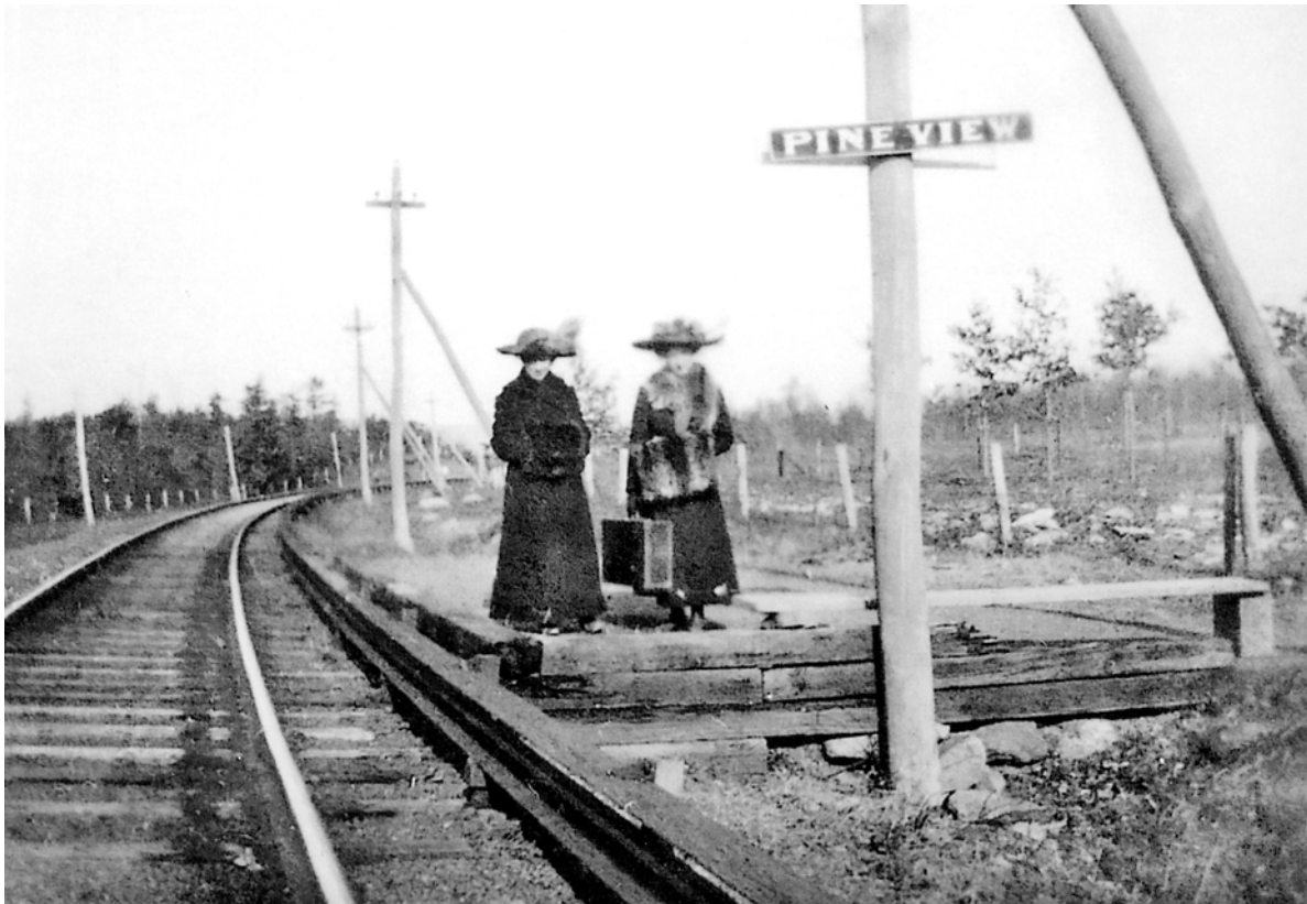
A humble sign, earthen platform, and makeshift bench mark the location of the Pine View stop on the Wilkes-Barre and Hazleton Railway in this undated photograph from the early twentieth century. Passengers boarding interurban cars here—bound either for Wilkes-Barre and points north or Hazleton and points south—stepped over the shrouded “third rail,” which carried power to the cars’ electric engines. Joseph Tweedle Sr. Collection
