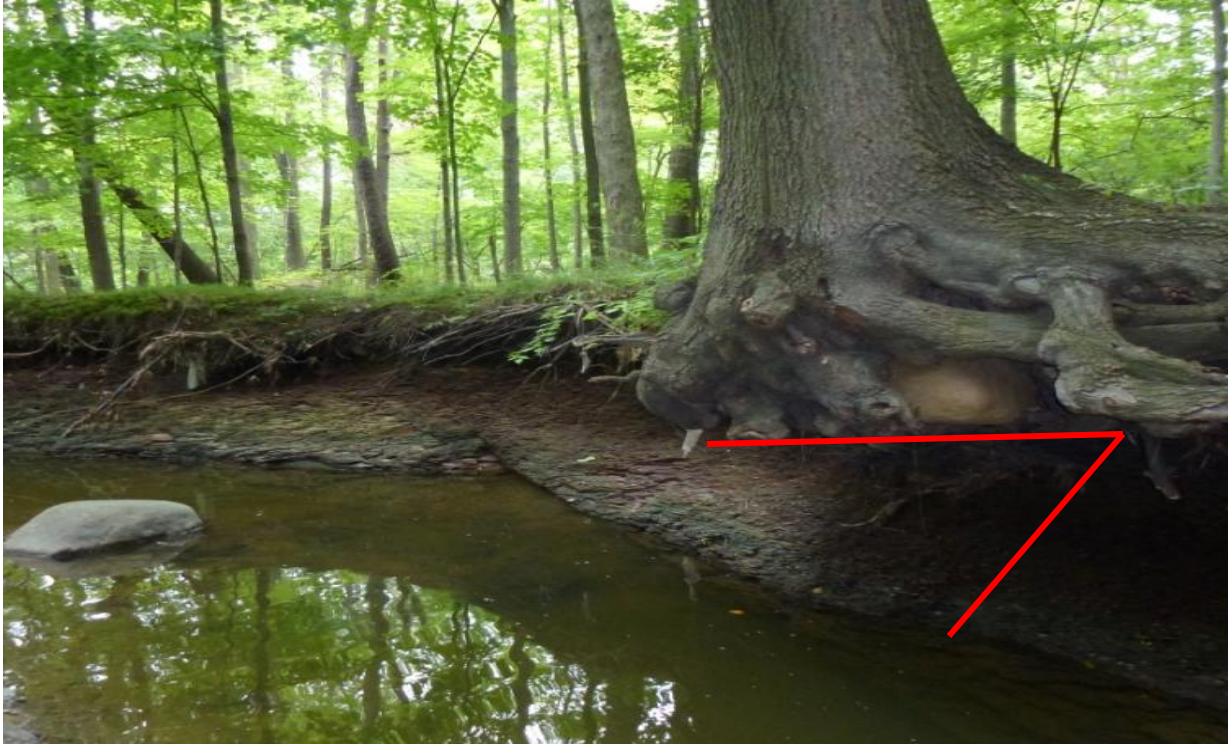
Figure 5: A bank with an extreme undercut.
