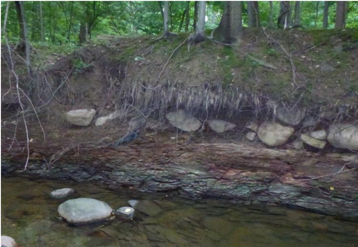
Figure 6: Boulders embedded in the stream bank, acting as surface protection.
