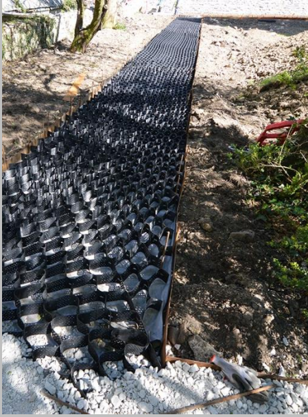
Sample image of a minimum impact6 pathway under construction
