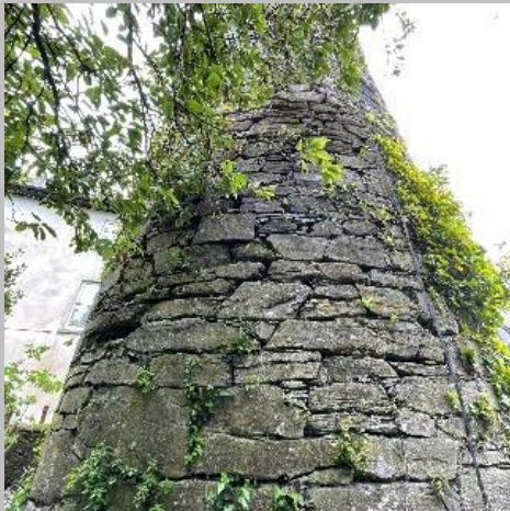
Tower base, southwest side. Note lightning protection to right
