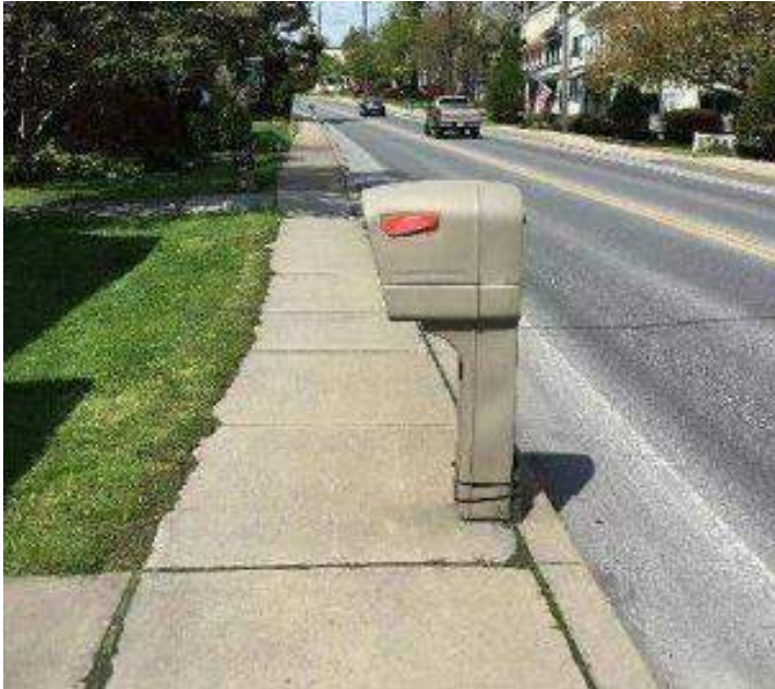
Sidewalk Obstruction - Mailbox
