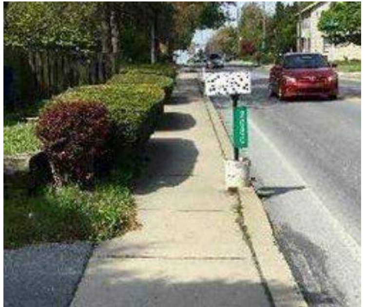
Sidewalk Obstruction - Vegetation
