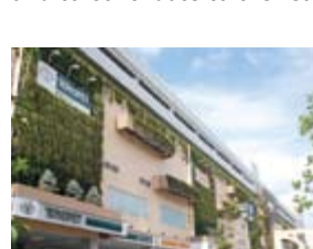
Wall greening of the north wing
