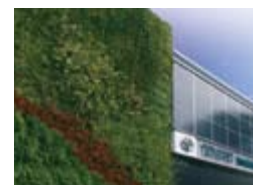
Solar power system and wall greenery
