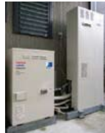
Solid Oxide Fuel Cell (SOFC) Cogeneration System for household use set up at a single unit home
