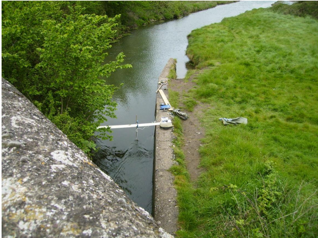
Figure 1. Main inlet/outlet channel where flow measurements were made in Cuskinny Lake during neap tides on 30 th April and during spring tides on 23 rd May 2012.
