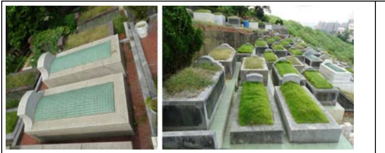
Figure 21. The visible upper layer of the tombs allow rain to enter, while the lower layers are sealed of. If the entire tombs is sealed, grass is emulated in Kaohsiung. No attempt to emulate a natural surface is made in Taipei, however, see images above.
