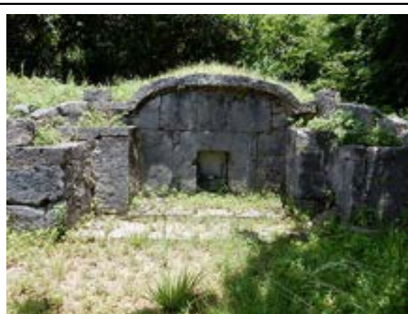
(b.) Izena, Okinawa, turtle-back style tomb. Raw building material, cut into large chunks and perfectly combined. Perfectly integrated in nature, it re-
