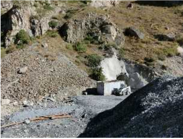
Site 1. Areas of the upper portal of the pressure conduit tunnel
