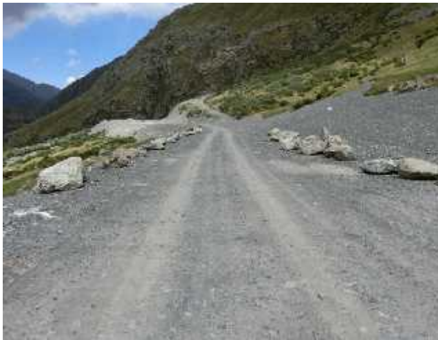
Site 6. Upper and lower slopes of the conduit way
