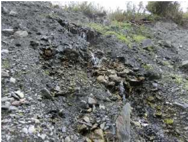
Site 3. The pioneer phase of vegetation restoration on the rocky soil after construction
