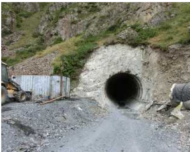
Site 1. Areas of the southern portal of the tunnel
