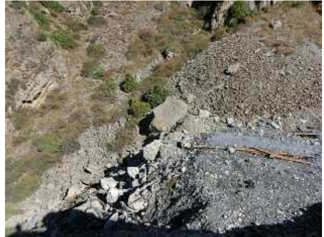
Site 1. Areas of the upper portal of the pressure conduit tunnel
