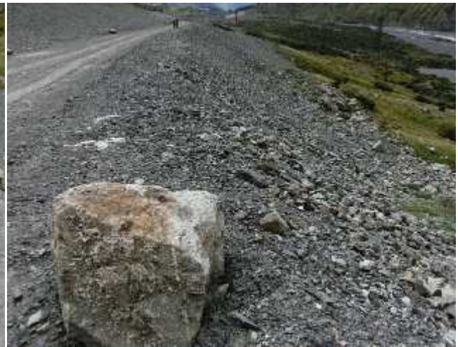
Site 6. Upper and lower slopes of the conduit way
