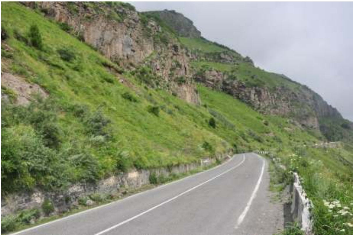
Picture 57: Polygon 151/7 is situated directly above the transit road. Shrub cover with 3 m distance to the road is the best solution for this site. Source: Roland Koeck
