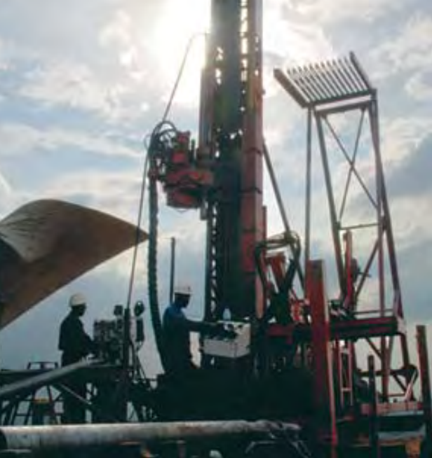
Drilling at the Kabanga nickel project, Tanzania
