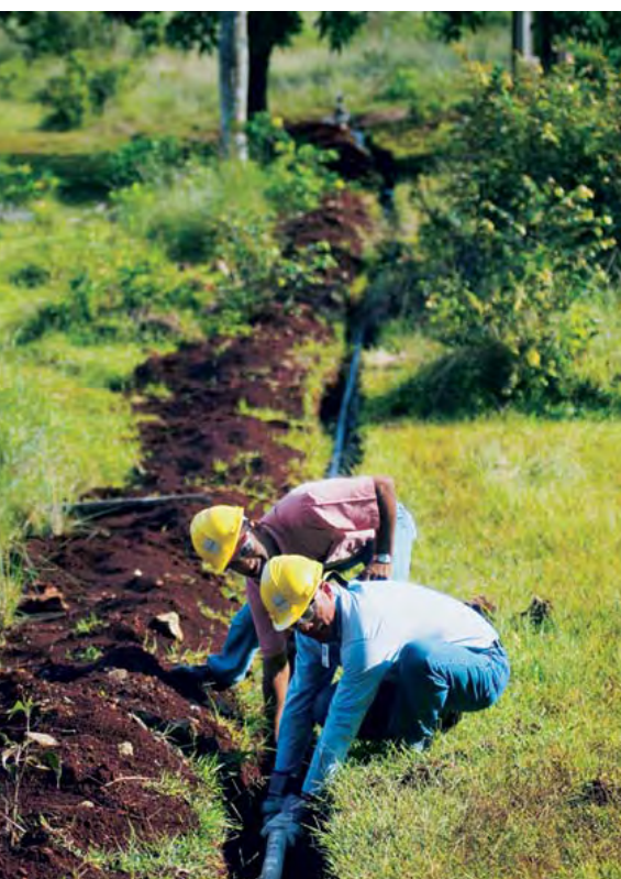
Testing water supply pipes at Falcondo, Dominican Republic
