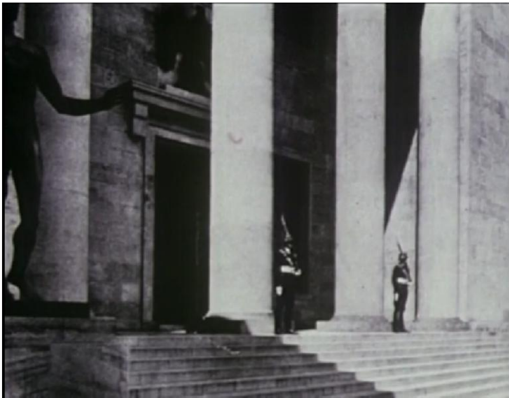
Figure VI-16b – Photograph of the portico in the New Chancellery’s Honor Court
