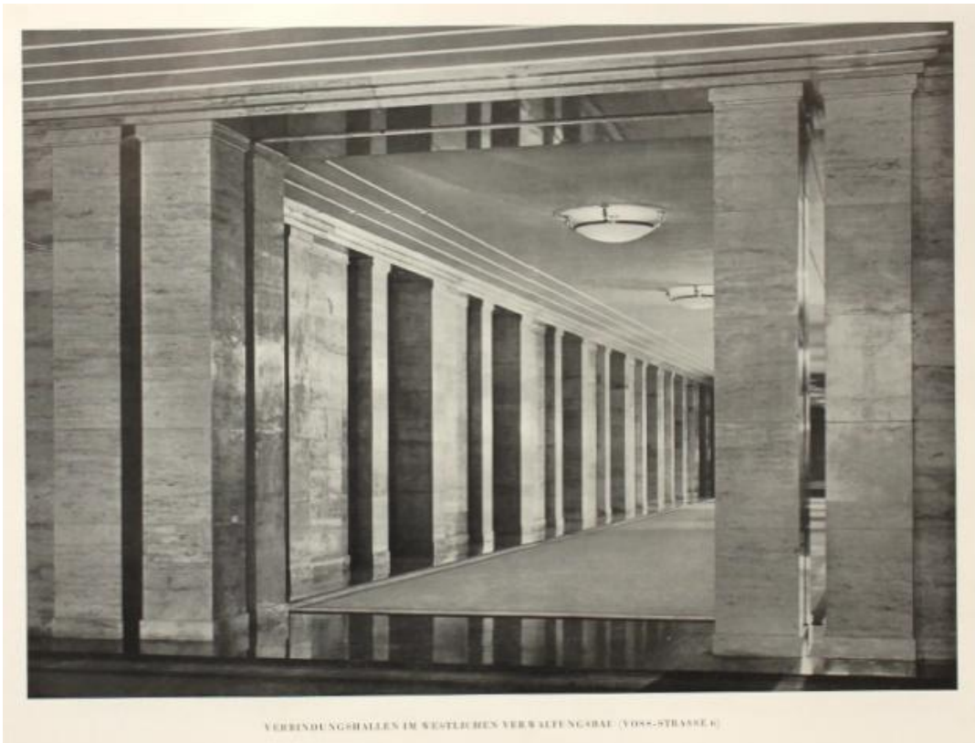
Figure II-47b – Corridor on the first floor of the Party Chancellery wing, direction of view unclear.
