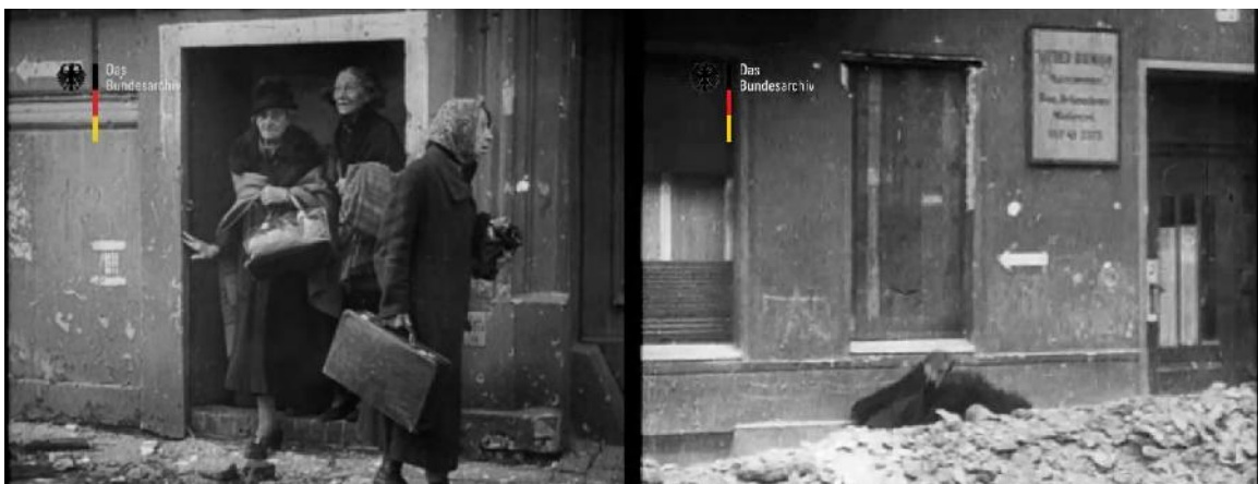
Figures IV-28a & b – Stills from das ende showing elderly German women exit from an air raid shelter (left), and a fleeing woman falling in the rubble (right)
