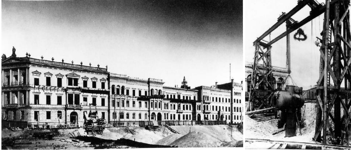
Figures II-12 & II-13 – Demolition for the re-laying of the Spree for the Great Hall's construction on Roonstraße ca. 1939. Source: Reichhardt and Schüche, pp. 154, 155.
