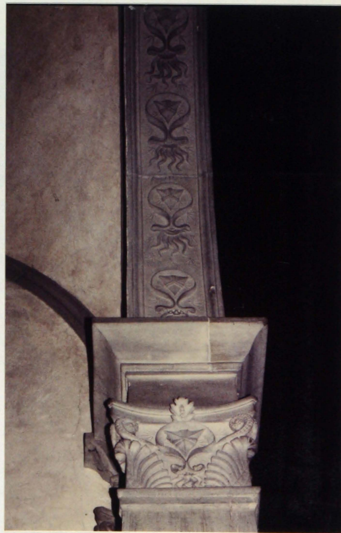
57. Tornabuoni chapel, Cestello, Florence: detail of the architectural decoration with the Tornabuoni device.
