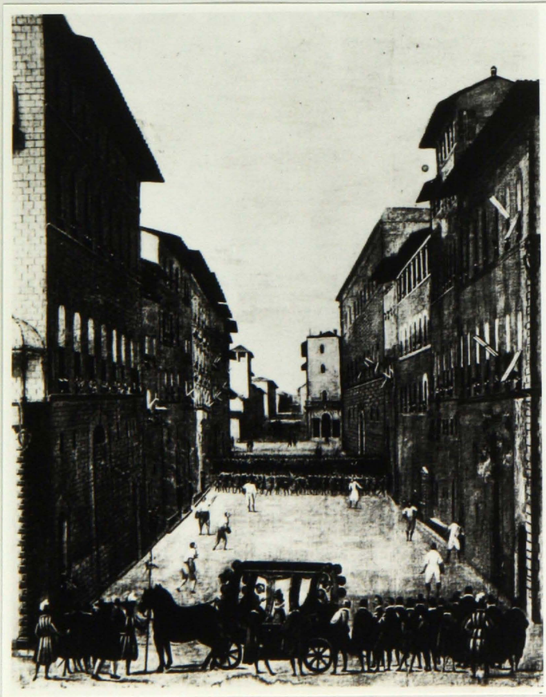
67. Anonymous: View down Via Tornabuoni showing Tornaquinci tower and loggia, 17th century, Giuntini Collection, Florence.
