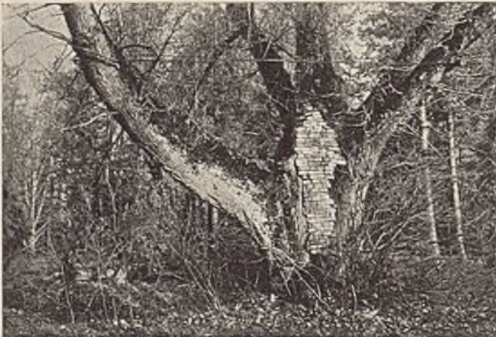
Ryc. 112. Stara lipa zamurowana i pościągana żelaznymi jarzmami. Cavity in Lime tree closed with bricks, and weak limbs secured by iron bolts.
